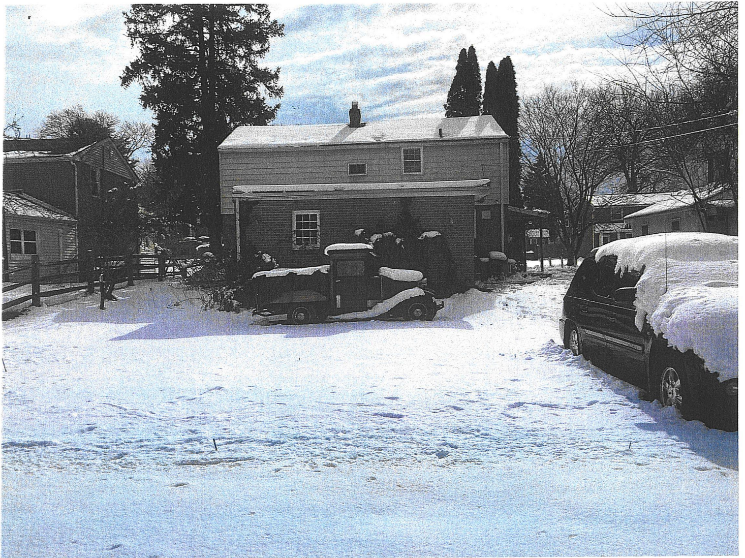
View of house from Backyard 4002 N. Warner Rd Lafayette Hill PA 19344
