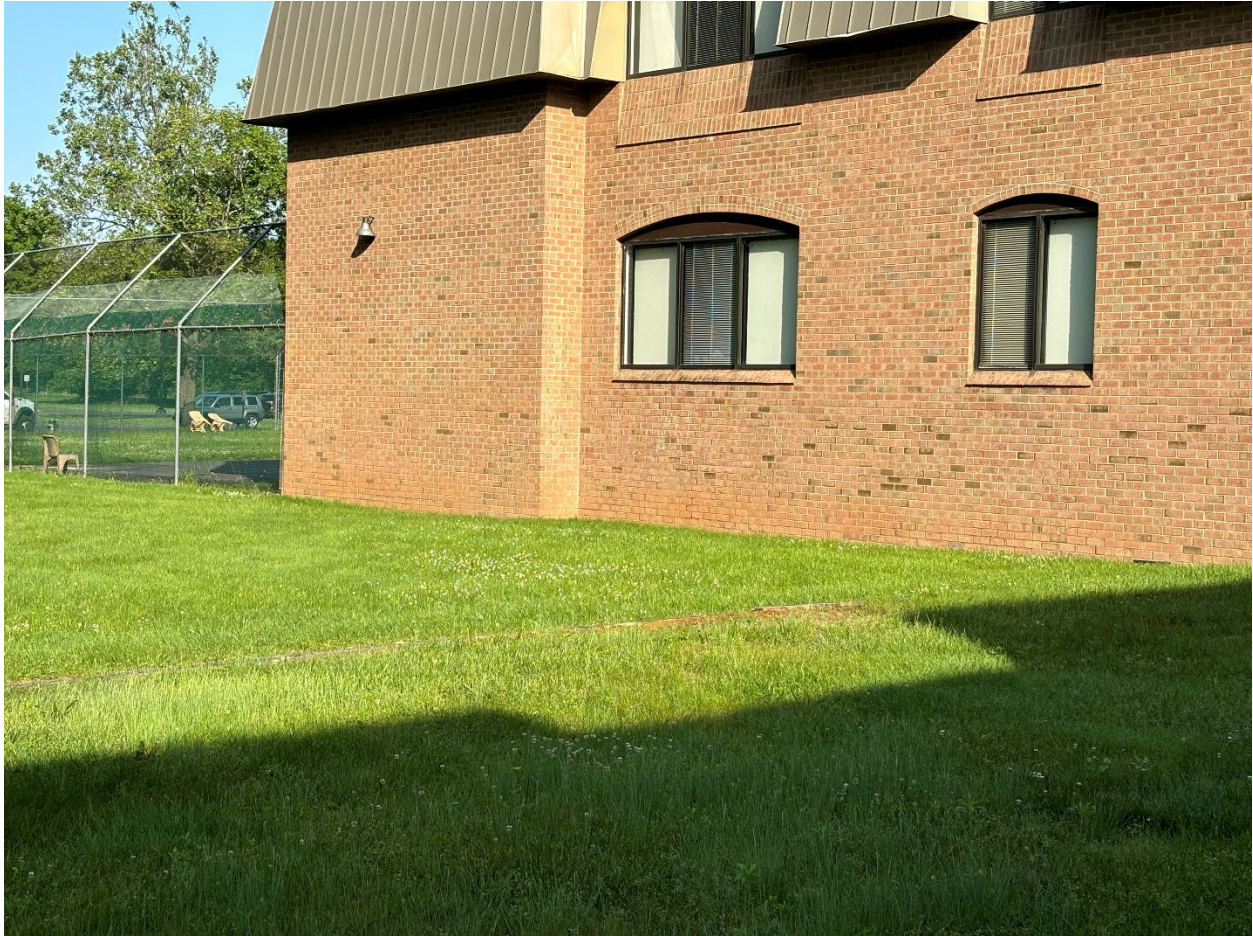
Southern building perimeter looking northwest at end of main courtyard fence.
