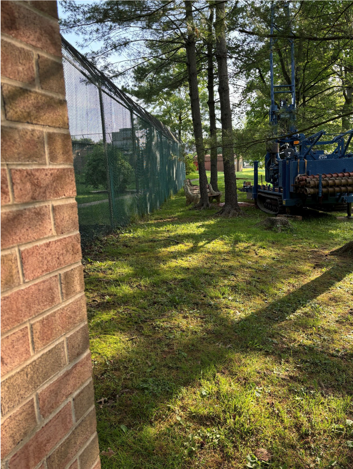
Southern building perimeter at beginning of small courtyard fence looking northeast.
