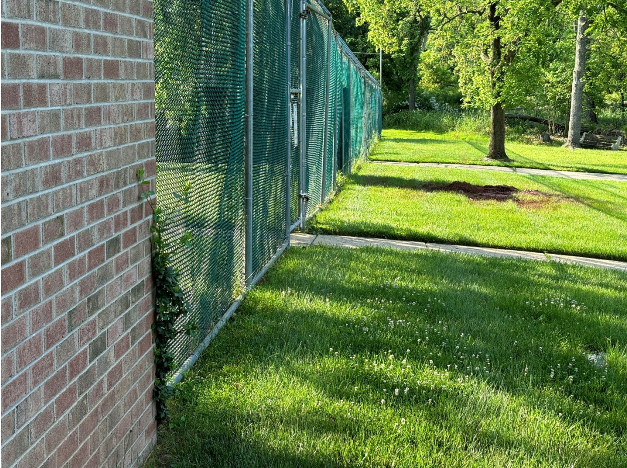
Western building perimeter at beginning of main courtyard fence looking southeast.
