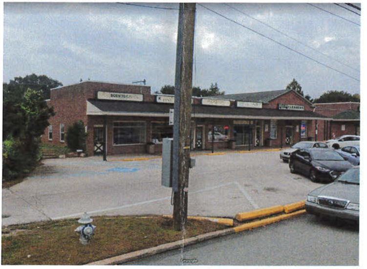
STREET ELEVATION PHOTO N.T.S.
