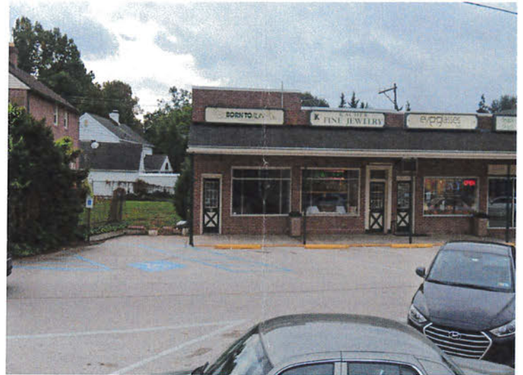
STREET ELEVATION PHOTO N.T.S.
