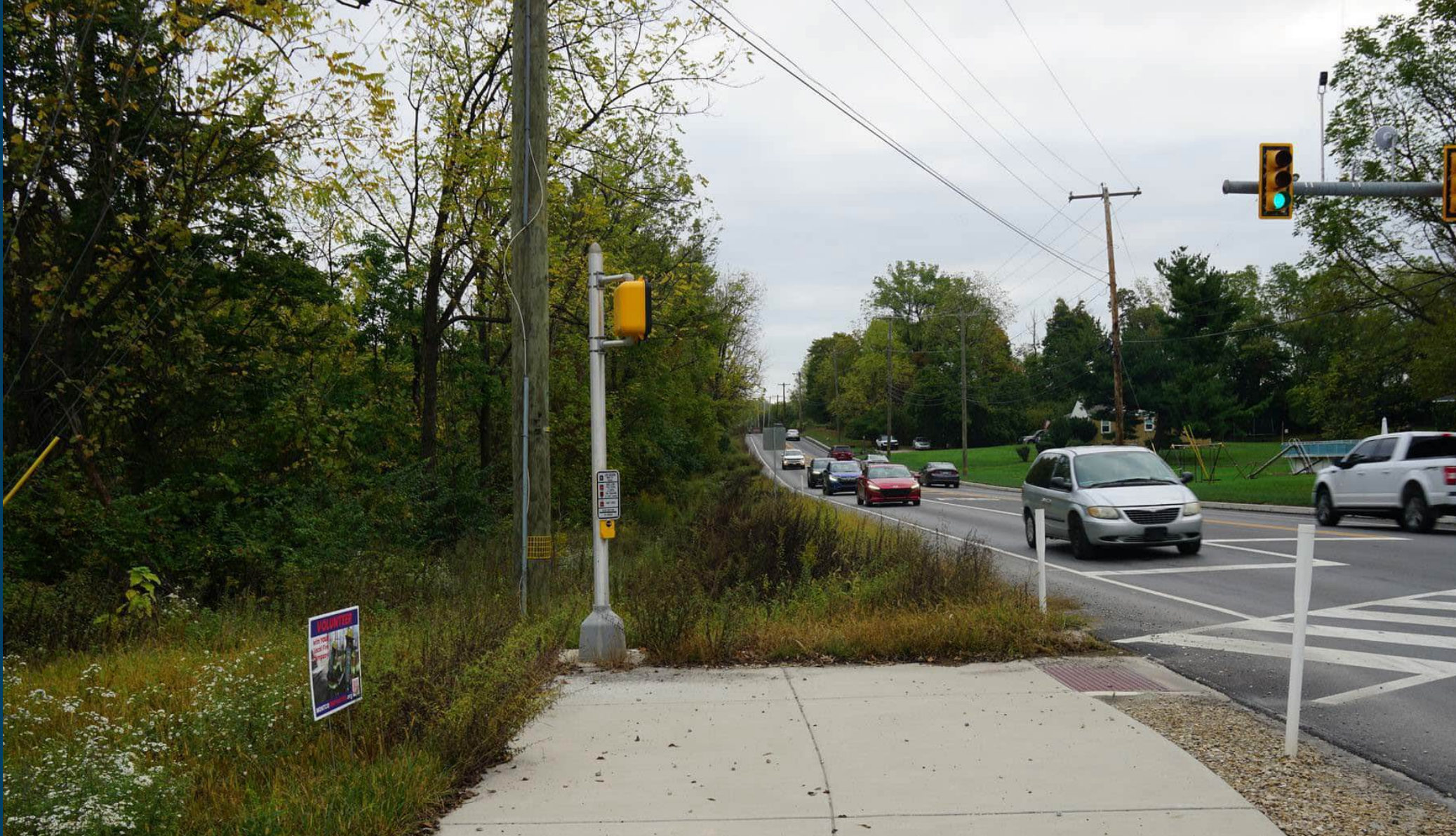
Photo 2: Joshua Road at Flourtown Road Looking North. Trail will be on the West Side of Joshua Road.
