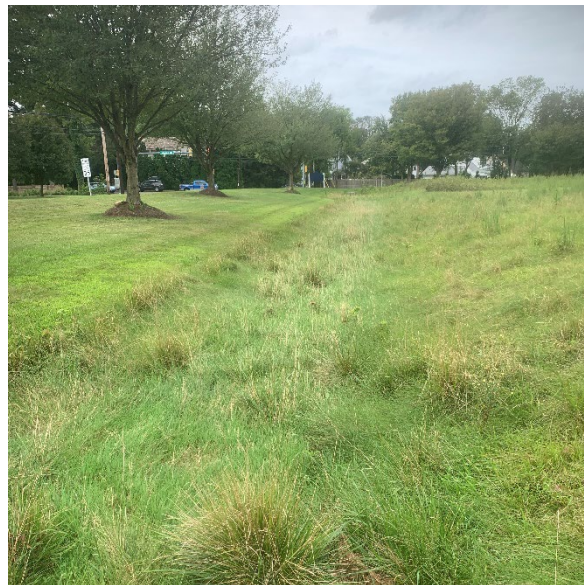
The existing swale features tall grasses and naturalized vegetation, which slows, filters and infiltrates water flowing off the meadow and the parking area.
