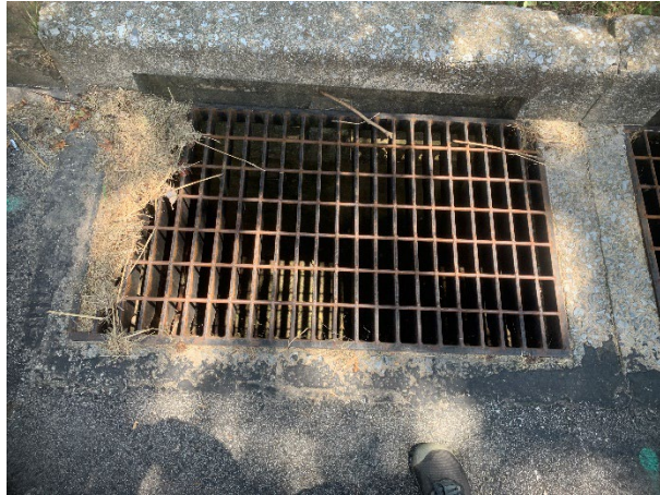
Grass clippings are washing into this inlet in the Joshua Knoll neighborhood, carrying nutrients into the basin and the watershed beyond.
