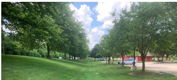
The turf swale is receiving runoff from the parking area and stormwater captured in other parts of the park. This swale could be naturalized to filter and infiltrate more stormwater and to provide more buffering between the park and the street.
