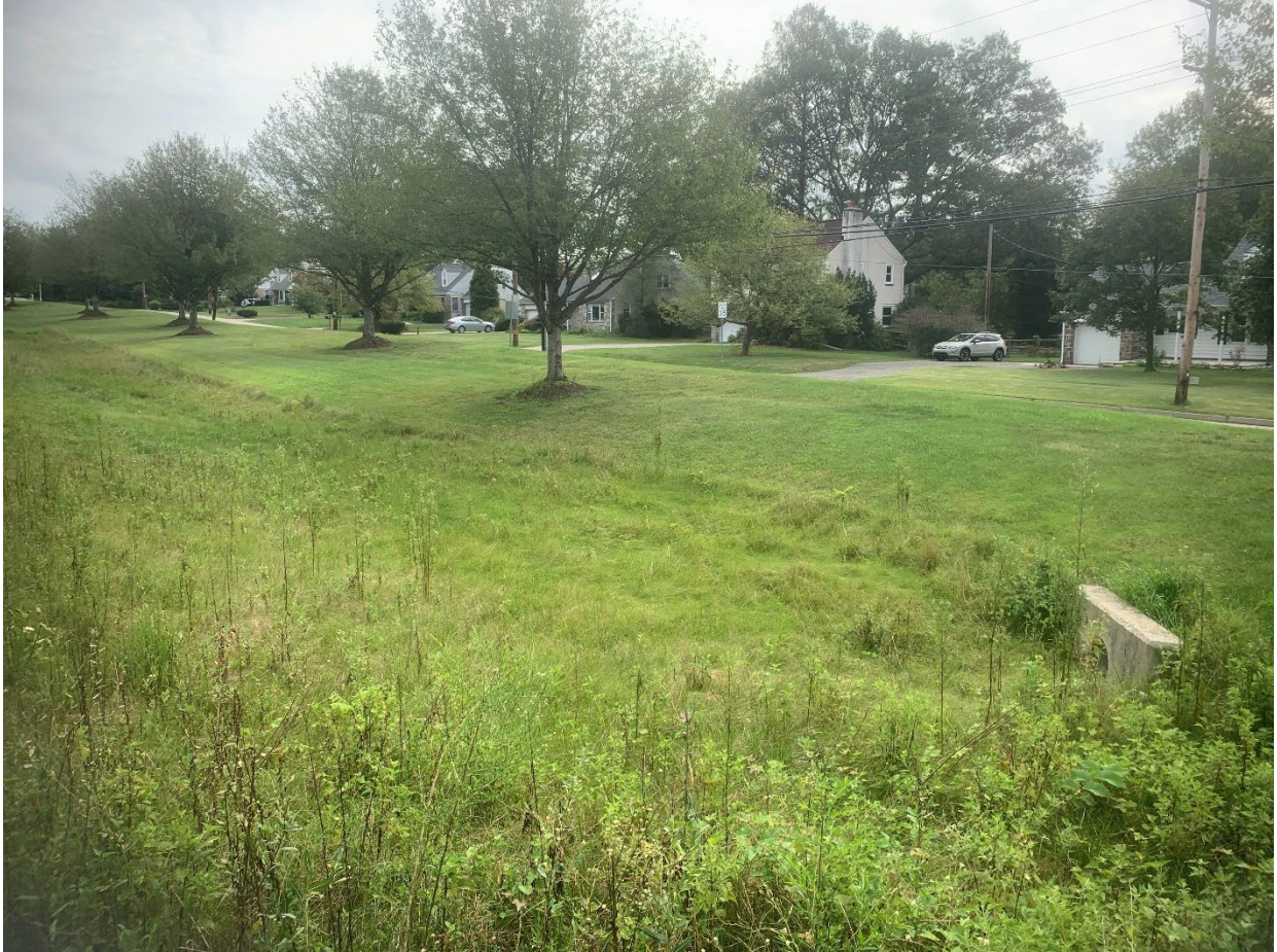
The vegetated swale acts as an extension of the meadow, resulting in a connected system of stormwater BMP's.
