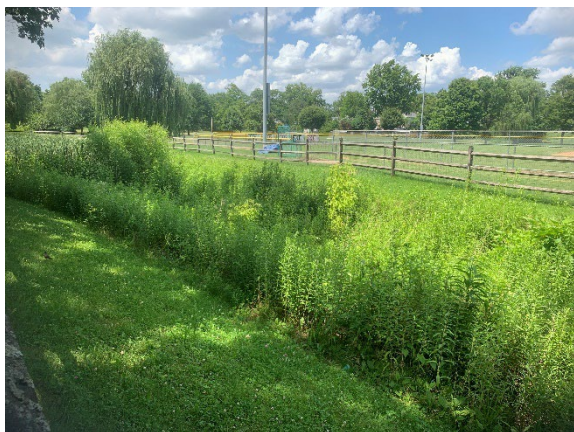
A portion of the stormwater system at Miles Park is naturalized. The same methods could be applied to the other swales and channels.
