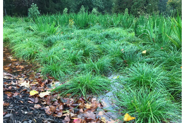
This rain garden at Natural Lands' Stoneleigh: A Natural Garden uses native plants to soak up stormwater running off the parking lot.
