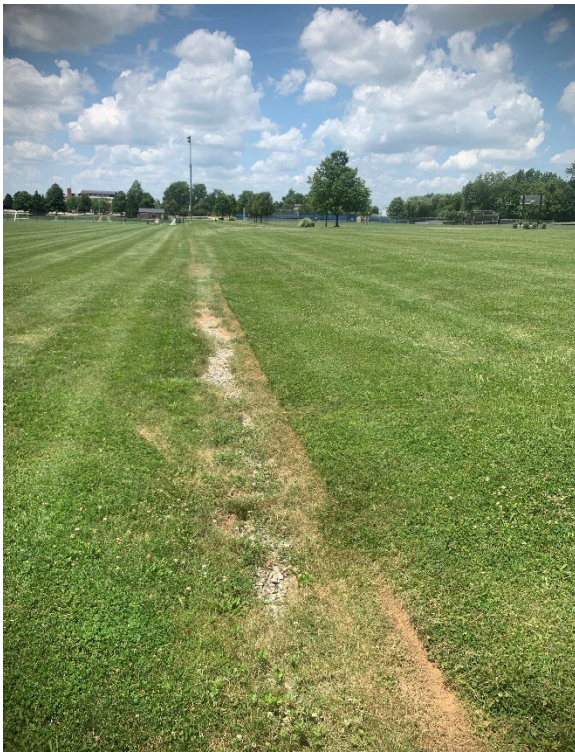
Swales are forming as storm water is collecting and eroding the fields as it flows to the basin. These areas could be improved with simple, easy to maintain plantings.
