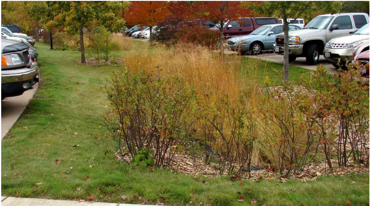
Through site visits and review of maps and aerial photography, we've identified opportunities from implementation of green stormwater infrastructure, like the planted island above, which captures and infiltrates stormwater.
