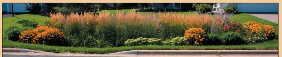
A dip in the curb allows stormwater runoff from the street to flow into the garden.
