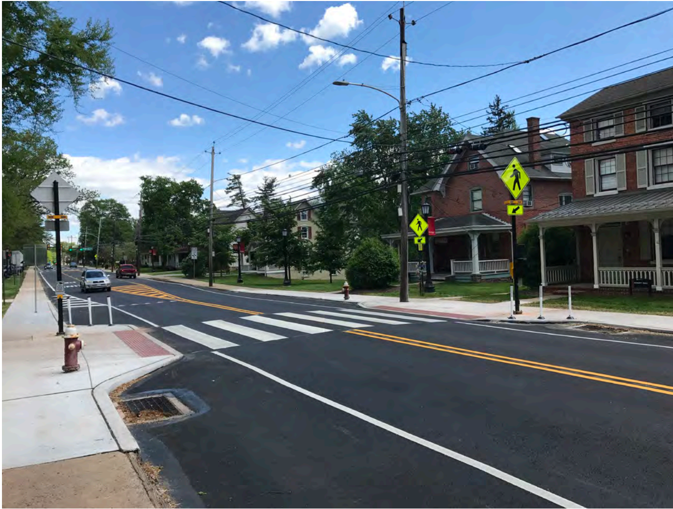
Pedestrian Crossing Improvements
